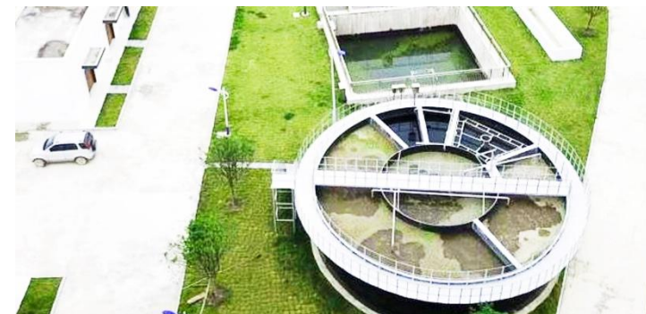
Urban sewage treatment integration AO project
