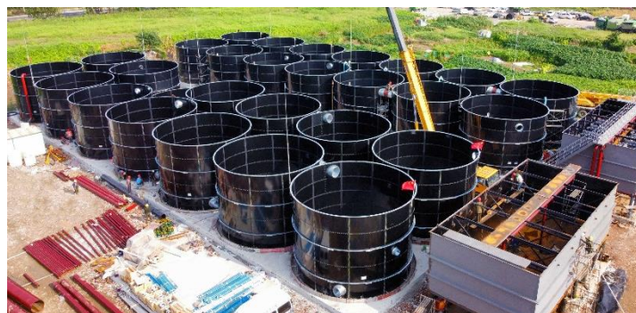
Jiangsu Wuzhong sewage project
