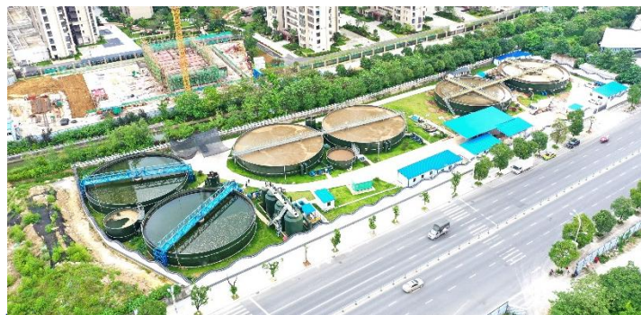
Guangxi Guilin sewage project
