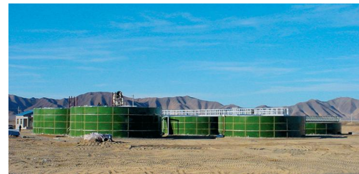
Jiuquan sewage project
