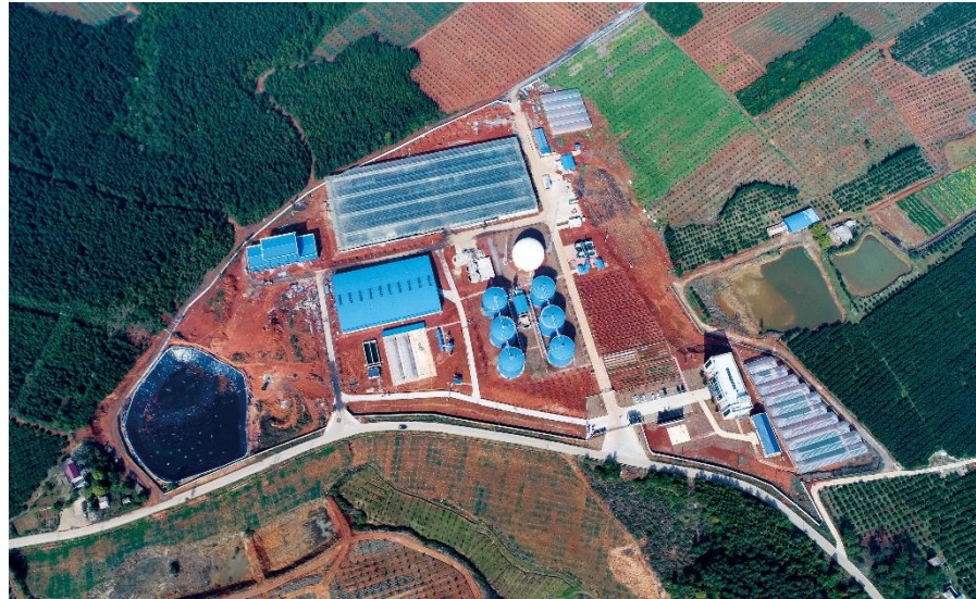
Xinyu centralized manure treatment plant
