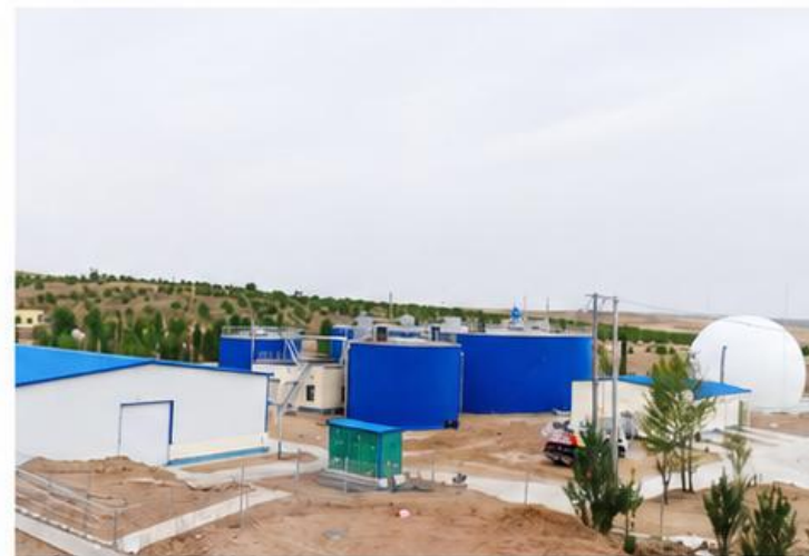
COFCO Chifeng pig farm project
