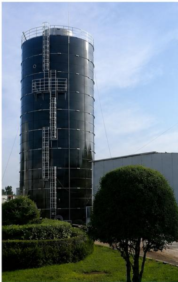
Pharmaceutical wastewater IC reactor
